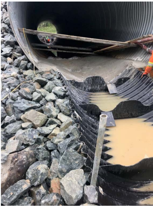
The flume was secured below the culvert with steel posts and rip rap.
