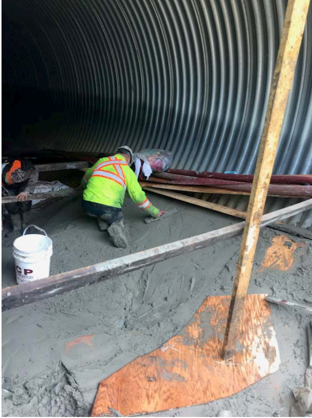
The damaged invert was repaired and the FISHCULVERT connection was sealed.
