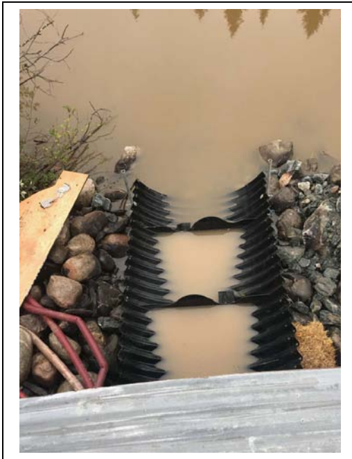
The flume was secured below the culvert with steel posts and rip rap.
